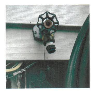
A cross connection is a point in a plumbing system where the potable water supply is connected to a non-potable source.
